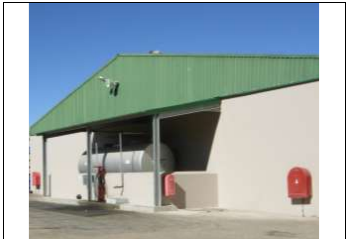
Photo 2.3: Example of an aboveground fuel tank within a roofed and bunded area at a Packhouse facility in the Sundays River Valley.
