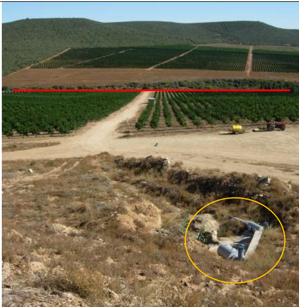
Photo 3.3: The irrigation pipe proposed to be installed on Portion 523 at the existing dam outlet pipe (yellow circle) and in the road along the existing citrus orchards, towards the DR01976 road (red line).
