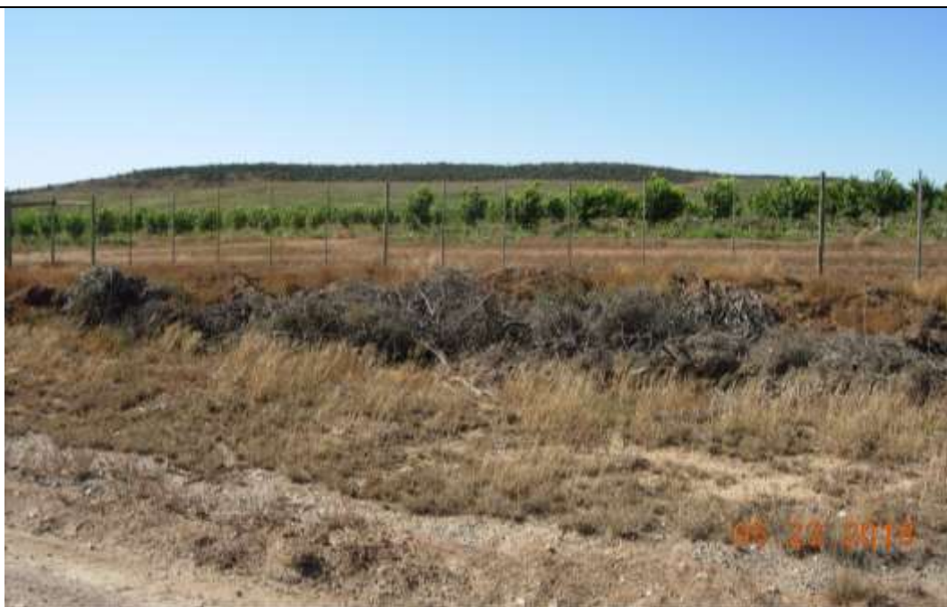
Photo 3.4: Example of irreversibly modified vegetation cover in the road reserve of the DR01976, where the irrigation pipe is proposed to be installed under and across the road from Portion 523 to Umgcambo.
