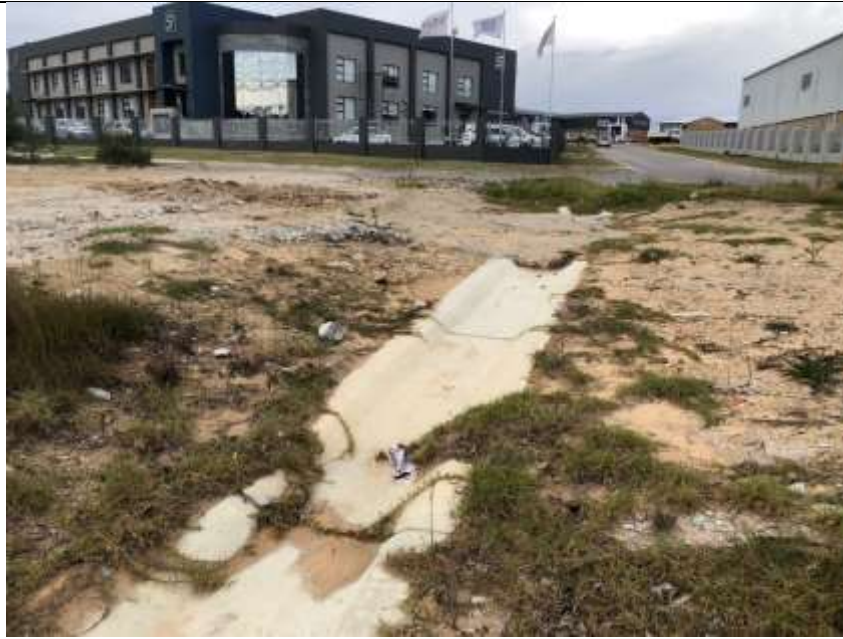
Plate 5.1: A view of the typical transformation that has taken place in the surrounding environment, showing high levels of sedimentation in the current storm water drains.
