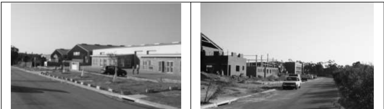
Photos of existing development adjacent to Phases 5 and 6, indicating the nature of development proposed.
