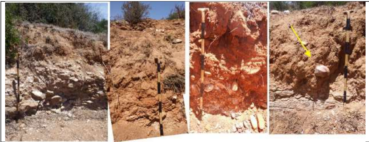
Figure 10.6: Weathered Sundays River Formation siltstones, capped by brown, sandy topsoils (A); thick, sandy alluvium with calcrete nodules (B); overlying a calcretised pebbly gravel (C); and a reworked core within superficial sandy soil (D). Scale 1 = 10cm.
