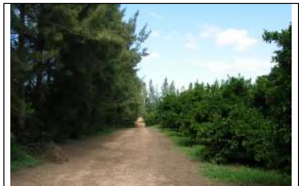
Photo 2.1: Example of internal service roads on an existing citrus farm in the Sundays River Valley.
