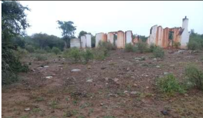
Photo 3.4: Example of irreversibly modified areas and ruined buildings associated with the historical settlement area.
