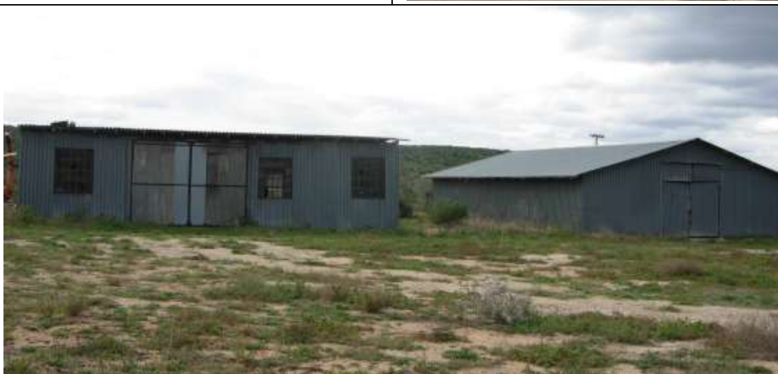
Photo 3.2: Existing farm structures on the Remainder of Portion 7 of Farm 98.
