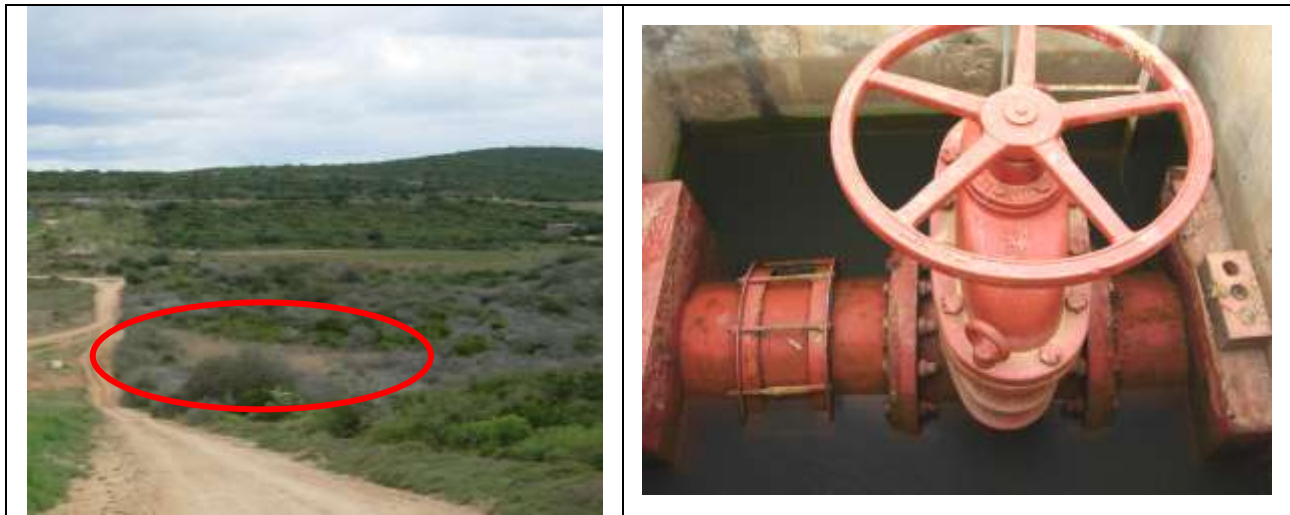
Photo 3.6: Wetland area adjacent to the southern boundary of the Remainder of Portion 7 of Farm 98. The wetland possibly results from a potential leak in the DWS dam on Portion 10 of Farm 98 (excluded from this assessment), or from a leak in a water pipeline with runs adjacent to the southern boundary of the Farm (pictured right).
