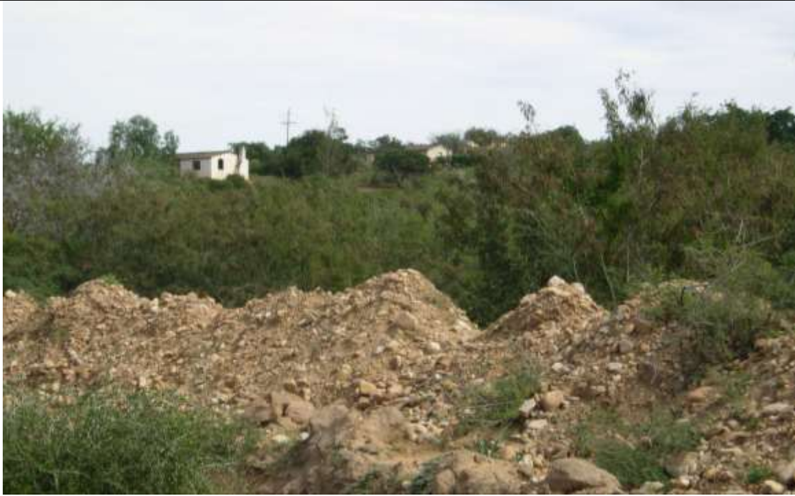
Photo 3.1: Looking towards the western boundary of the area under assessment: the trench that has been dug along the eastern boundary of the area under assessment. Ruined buildings can be seen in the background.
